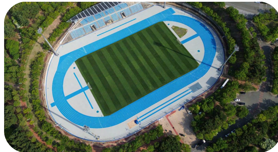
<Daegu Auxiliary Stadium - Inside View>
